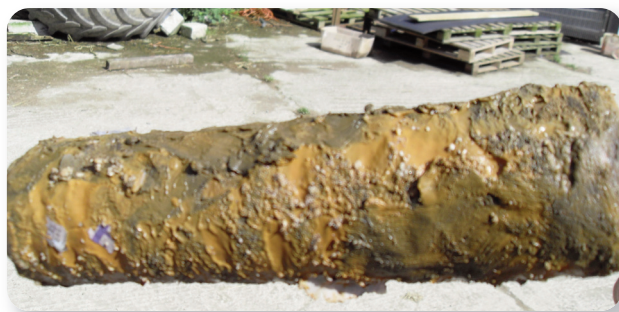
A water filter clogged up with sedimentation
